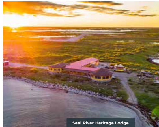
Seal River Heritage Lodge
